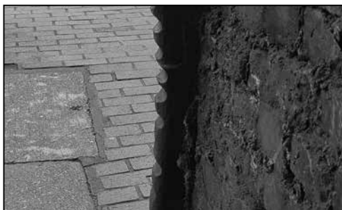
Wharf Road Bridge showing rope grooves
